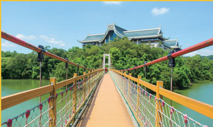
細茅埔吊橋 Ximaopu Suspension Bridge
